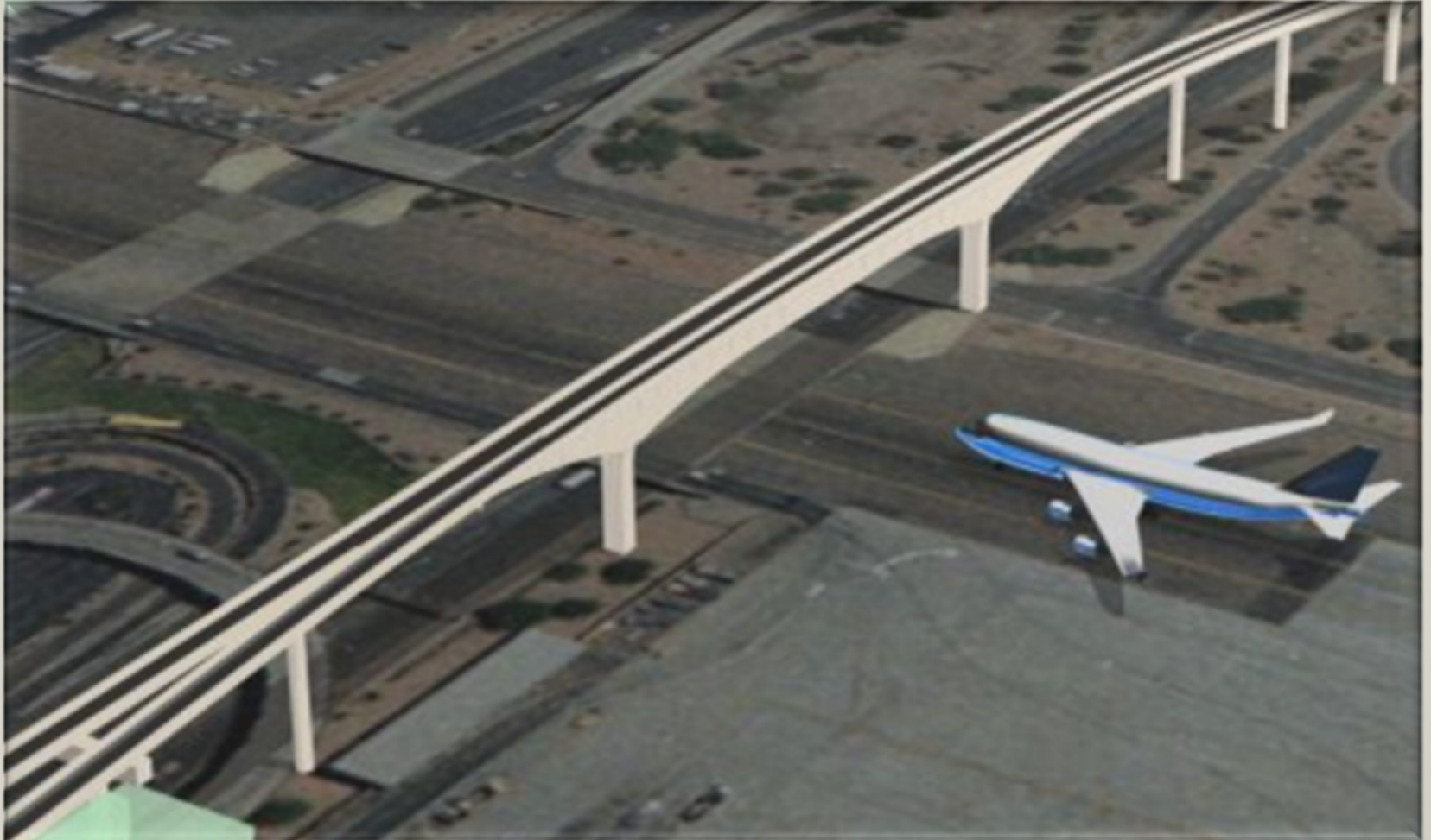
Post-Tensioned Concrete Box Girder
